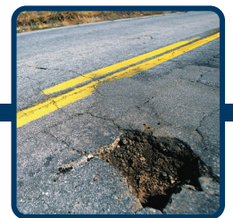
POTHOLES/DAMAGED PAVEMENT
